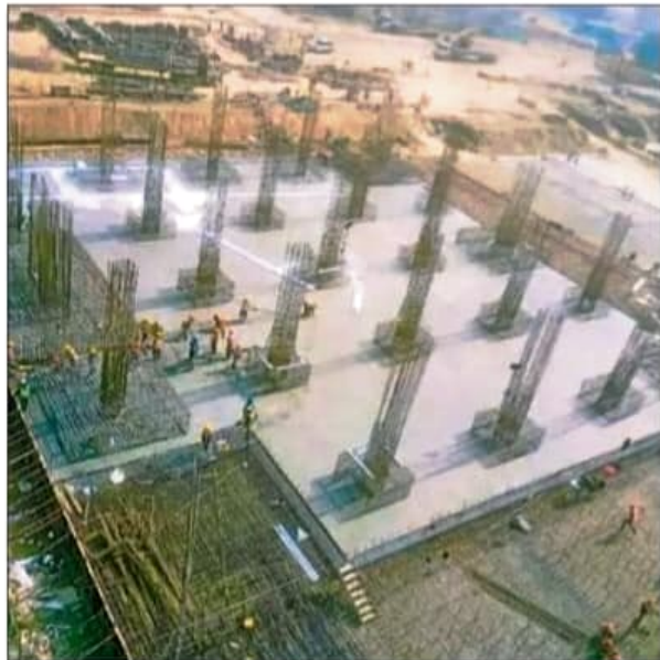
Work underway at the upcoming Noida airport in Jewar. HT PHOTO
